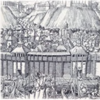
Kyiv harbour in Pochaina, the reconstruction
